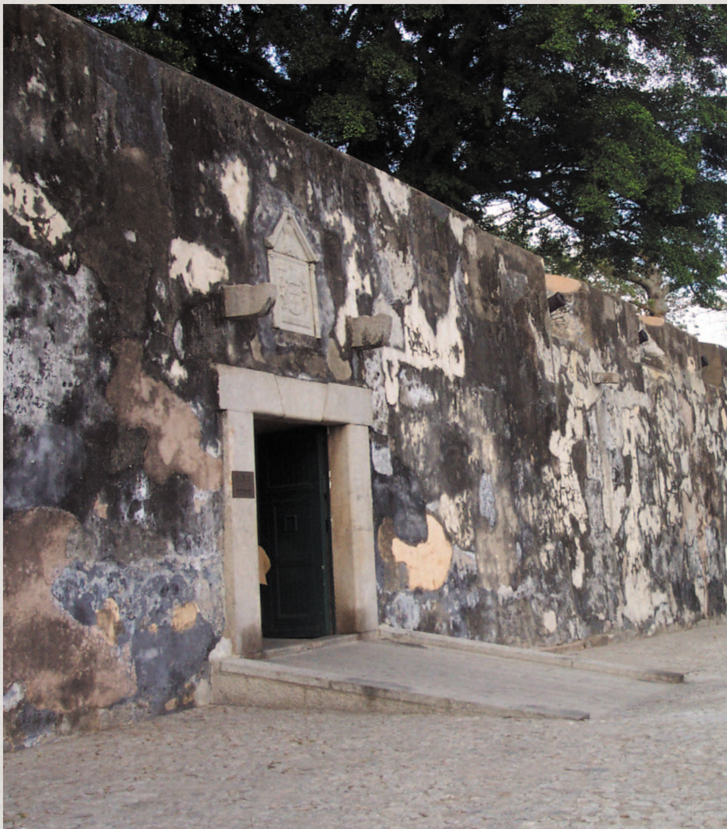
Fig. 2. South face of the Monte Fort.
