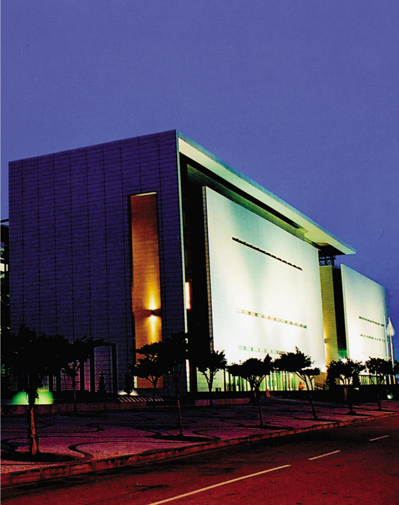
The modern and sophisticated façade of the Macao Museum of Art (MAM). Photo by MAM.
