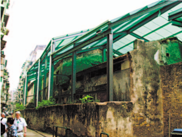
Fig. 5 - Restoration work at the Mandarin's House, Macao (10 September 2002).
